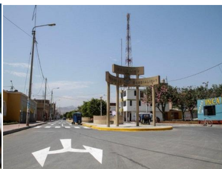
New roads and sidewalks in Huarney.
